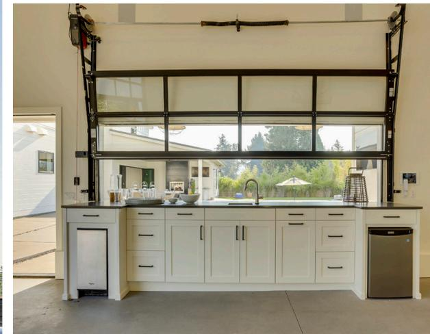
High-lift tracks go up the wall instead of overhead for a clean, open feel. Frosted glass provides privacy or clear glass admits natural light as desired.
